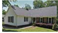
Gardner Park! Master down! So much space! So much style! $149,900
